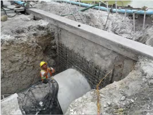
Repaired and reconstructed six culvert crossings with significant erosion problems, improving safety, stormwater management, and reducing pollutant runoff.
