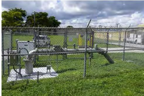
Raw Water Rehabilitation Project, reconfigured four (4) raw water wells to be above 100-Year Flood Levels and replace all mechanical, electrical, and control equipment. This projects protects the water supply from flood water and makes the equipment more accessible for maintenance.
